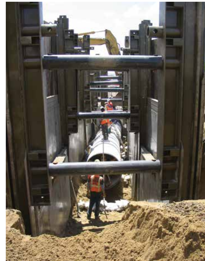
(left) Point of the Mountain Aqueduct—completed in 2007—was a challenging 12-mile-long culinary water pipeline connecting Little Cottonwood Treatment Plant with Point of the Mountain Water Treatment Plant. (right) Geneva Rock’s innovative Point of the Mountain conveyor belt system was built from 2012-14, officially going online in May 2014.
