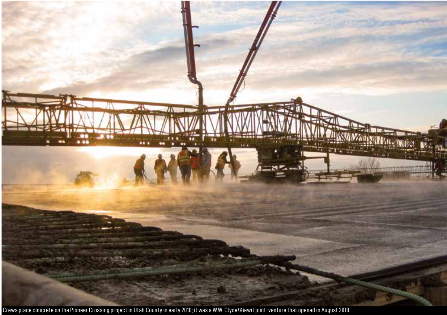
Crews place concrete on the Pioneer Crossing project in Utah County in early 2010; it was a W.W. Clyde/Kiewit joint-venture that opened in August 2010.
